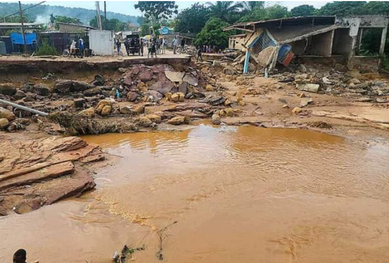
Debris from what was a bridge over the Ndjili River is shown in the aftermath of severe flooding in Kinshasa, Congo. With the bridge washed away, worshippers are unable to reach Lemba Imbu United Methodist Church, which also was damaged by floodwaters following torrential rains on April 5. Photo by the Rev. Fiston Okito, UM News.
